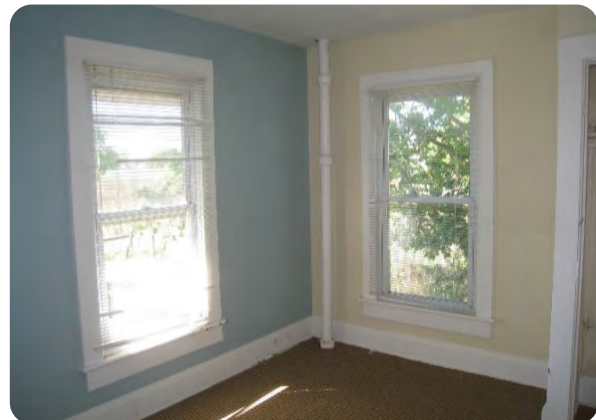
Existing bedroom (exposed vent pipe)
