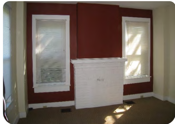
Painted brick fireplace used as a furnace vent
