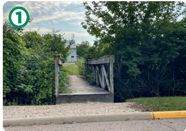
1 Bridge, Daniel Wright Elementary
