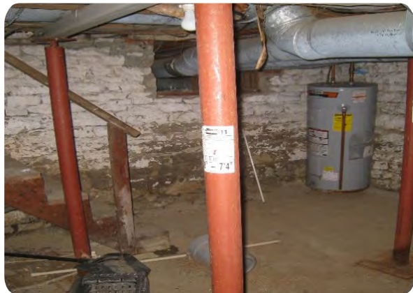
Shoring posts and older water heater
