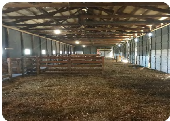
Existing barn interior
