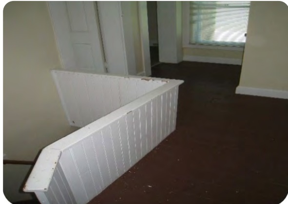
Existing stairway guard-wall assembly
