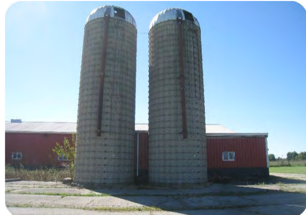
Building 2 - North Elevation at silos
