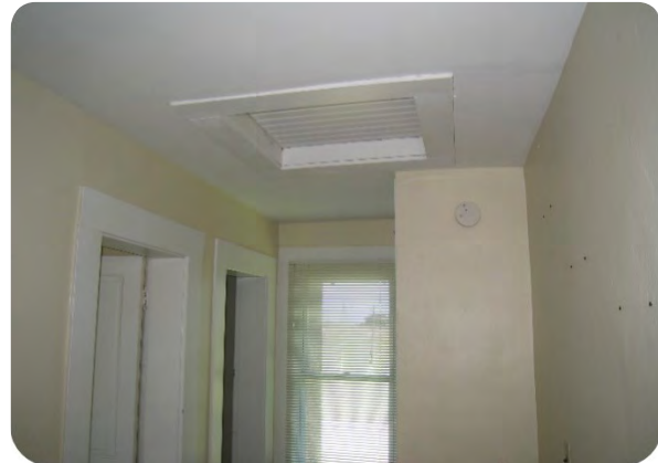
Existing attic access panel in hallway
