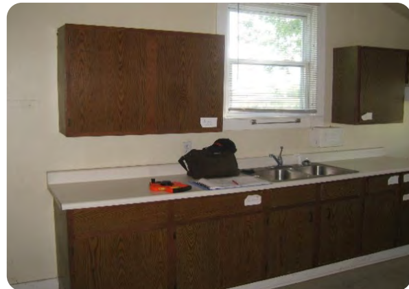
Existing kitchen sink and counter
