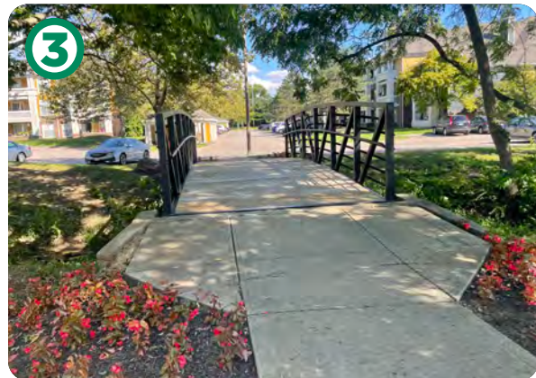
3 Bridge, Sterling Place Apts.
